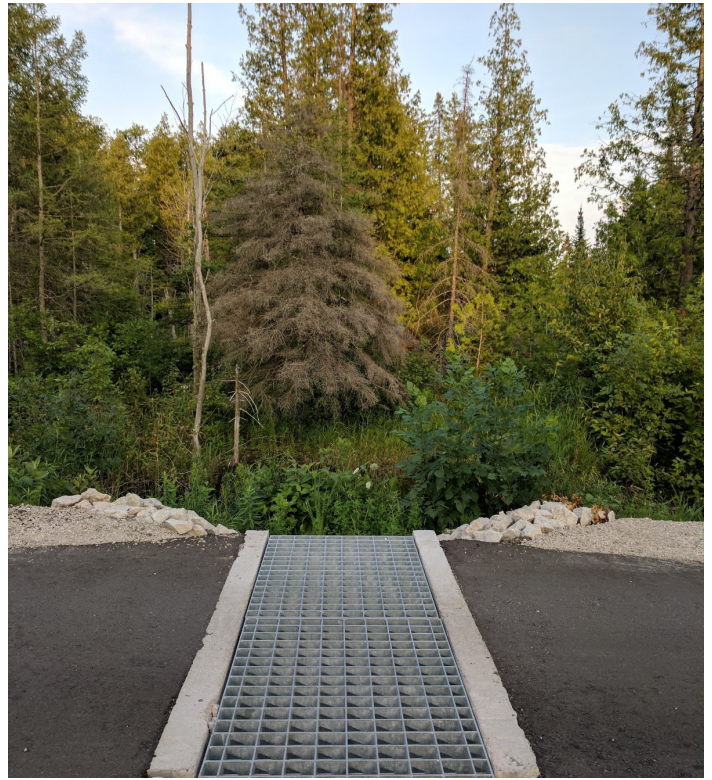
Wildlife mitigation 'daylighted' crossing structure, Ontario
