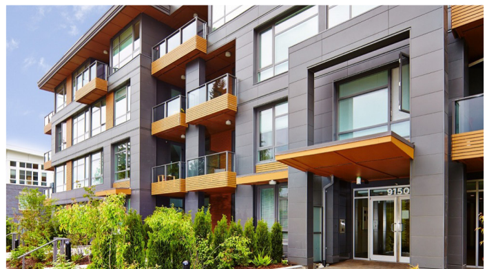
UniverCity 'Veritas' Energy Efficient Construction, Simon Fraser University. Source: Porte
