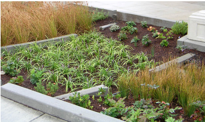
Bioswale along streetscape. Source: National Association of City Transportation Officials
