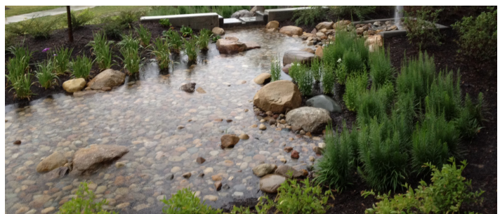
Rain garden stormwater management at Bridgestone Americas, Akron, Ohio. Source: Environmental Design Group
