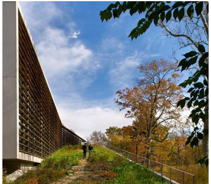
Nature-inclusive design with preserved mature trees and integrated green roof. Centre for Global Conservation. Source: Architectural Record
