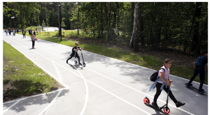
500m multi-use path improves cycling and pedestrian accessibility, Genk, Belgium Source: erwinvanamstel.com
