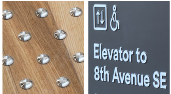
Calgary Central Library coordinated its public realm and building design with established standards of care in terms of public accessibility. Source: Calgary Library
